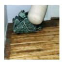
Before the sanding procedure, use a punch to countersink any raised nails. Then start with the roller sander and more-or-less coarse sandpaper, depending on the condition of the floor (old paint, adhesives, etc.). Use the edge sander to sand the remaining surfaces.
